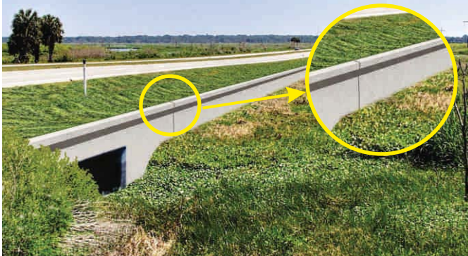
Figure 9.7. An outward lip in the wall for directing animals, especially snakes, towards underpasses.
